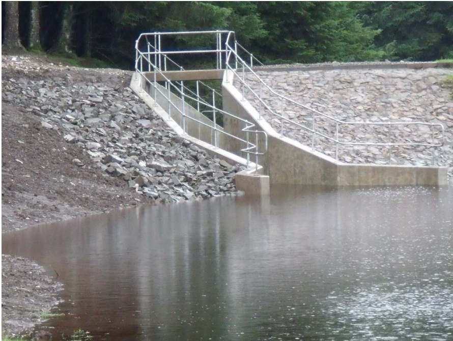
Discontinuance Works (2009) 43,000m 3 – 23,750m 3 capacity
